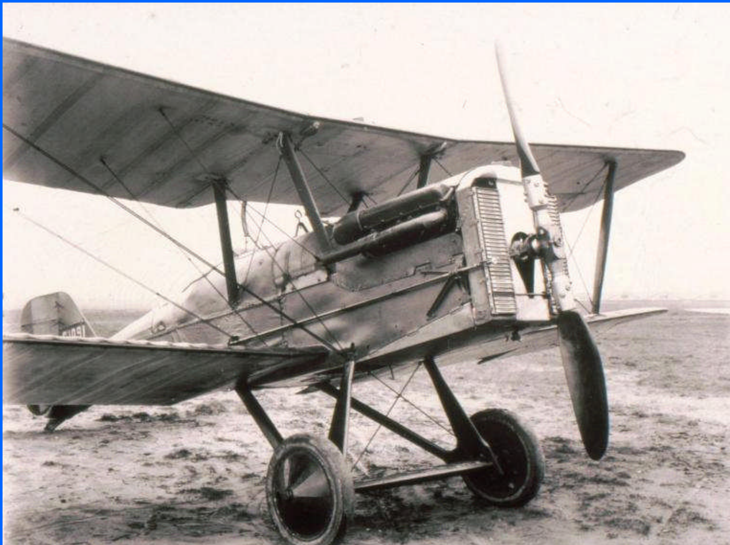
Lynam's Experimental VP airscrew on SE-5a - c.1917
